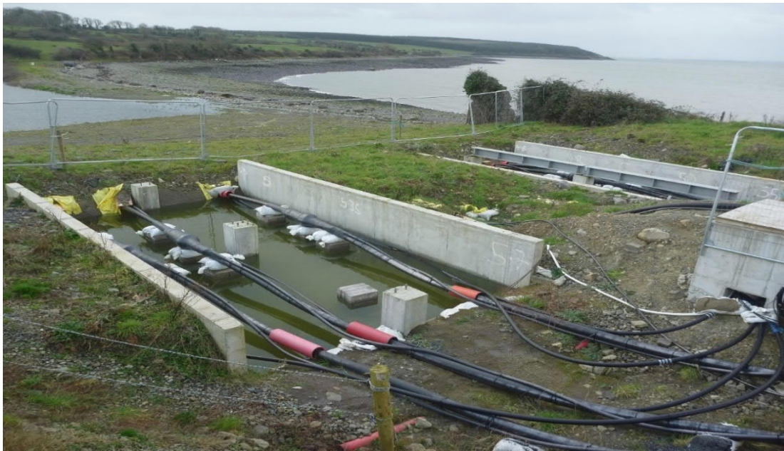
Figure 2.6: Typical Transition Joint Bay Before Final reinstatement
