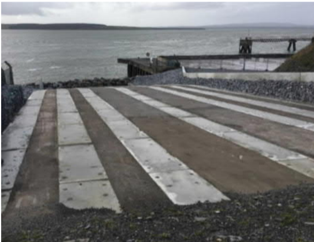
Figure 2.7: Typical Transition Joint Bay following final reinstatement
